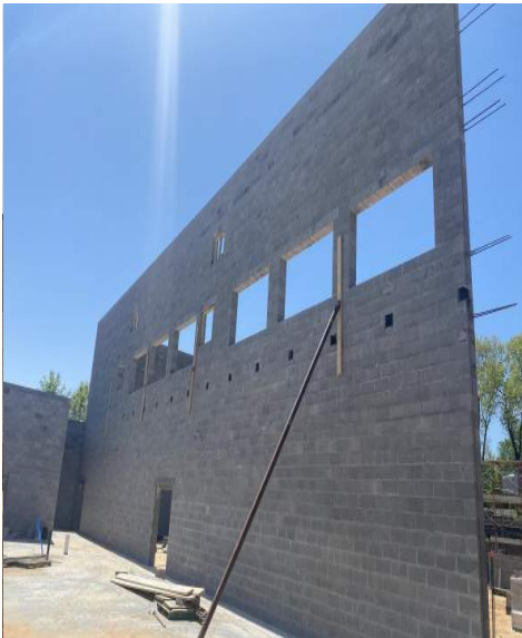
CMU Load Bearing Wall being installed
